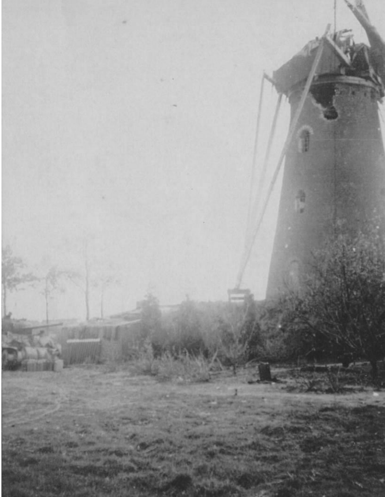
Gilbert's tank beside the heavily damaged mill
